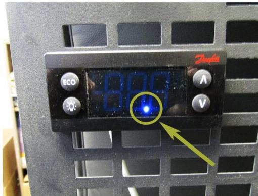
To turn the refrigeration back on, all you need to do is press and hold the lightbulb button for a few seconds until the chiller turns back on, and voila! The refrigeration is up and running again.
