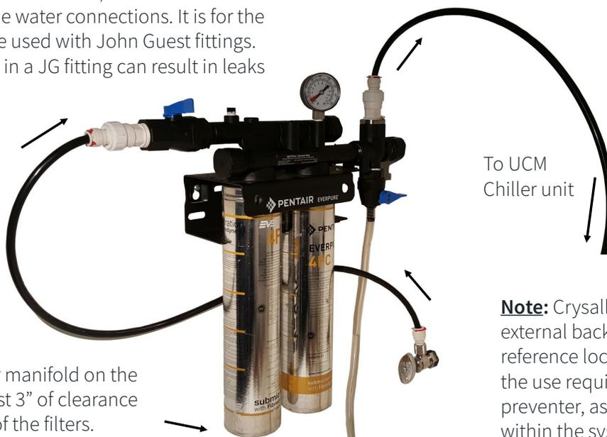
Mount the filter manifold on the wall with at least 3" of clearance at the bottom of the filters.
