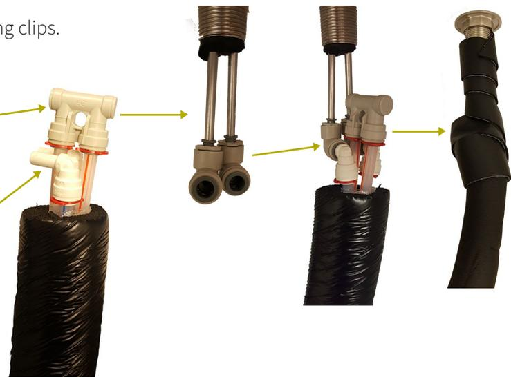
**Step 4:** Once assembled, connect the stem end of the plug in elbow fittings to the super seal fittings on the tower. Connect the blue striped tube to left faucet tube for sparkling water. Natural to still chilled water. If using a 3-valve tower, run a separate hose from the filter to the 3rd tube for ambient water. After testing the system for leaks, wrap all exposed hoses and fittings with the insulated tap found in the UCM install kit.
