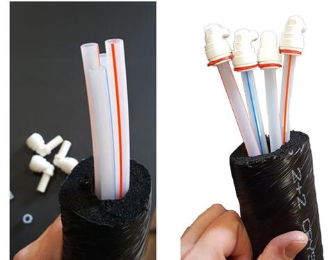
**Step 4:** Connect the hoses to the outlets:
